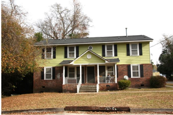
SITE – Summit at Belmont Apartments 5703-5716 Randall Avenue, Columbia, SC Typical existing structure on site Facing east from Oakland Avenue Randall Avenue Extension is to right of building
