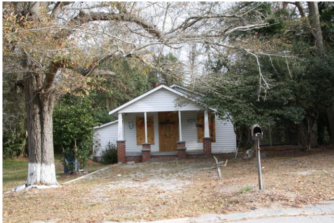
SITE – Summit at Belmont Apartments 5703-5716 Randall Avenue, Columbia, SC Existing single-family home to be razed Facing east from Oakland Avenue Randall Avenue Extension is to left of home
